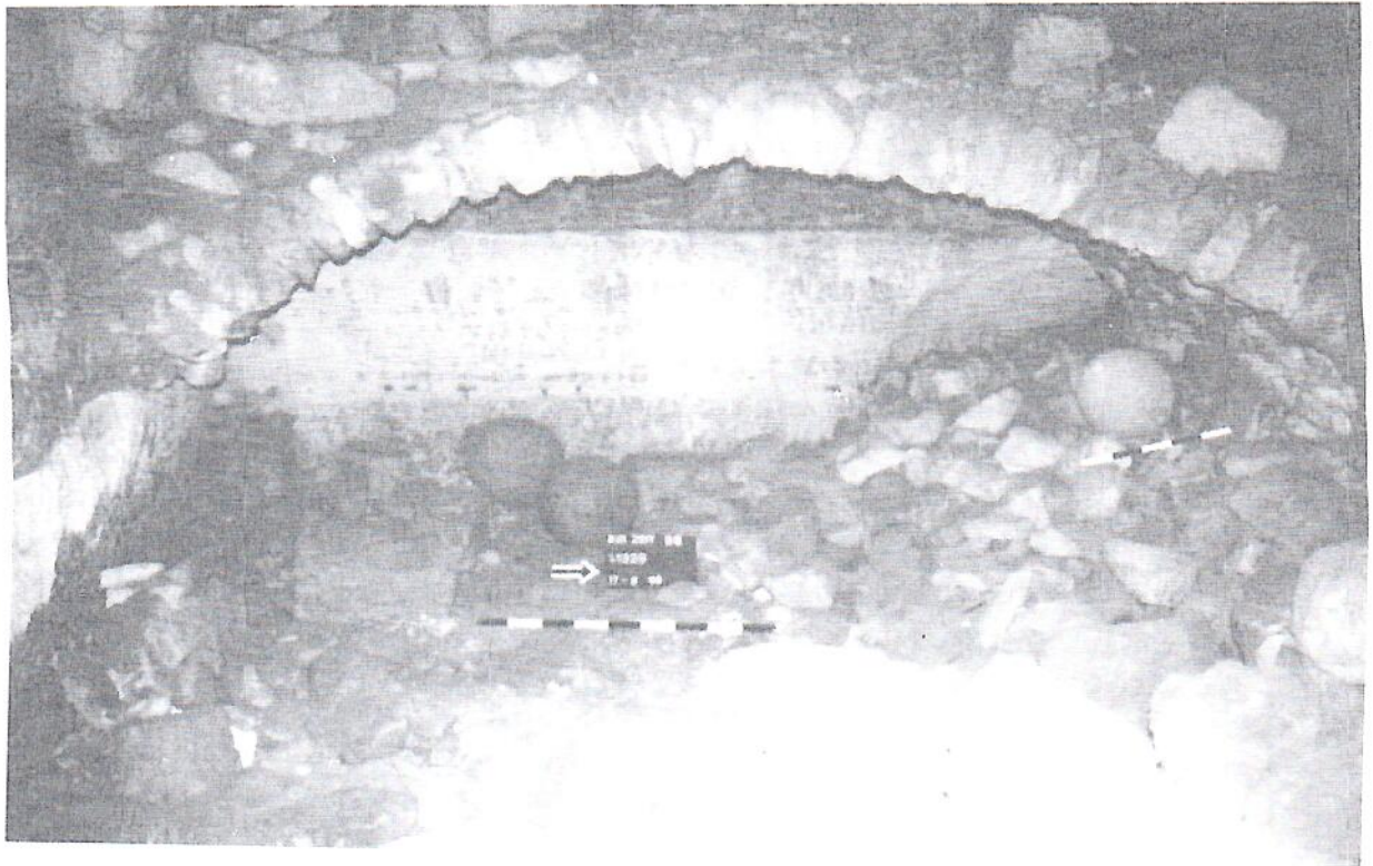
Fig. 8. Northern Hall: Northern Lower Room, Western Part
